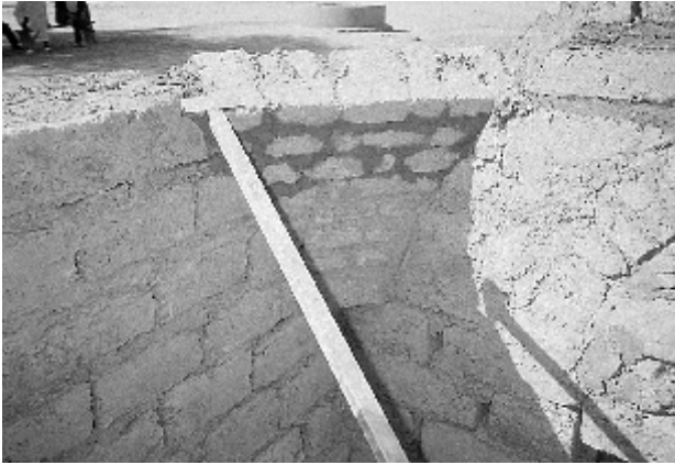
Fig. 11 The radial arm showing the placing of bricks in a pendentive, the lower part of the corner of a dome.
