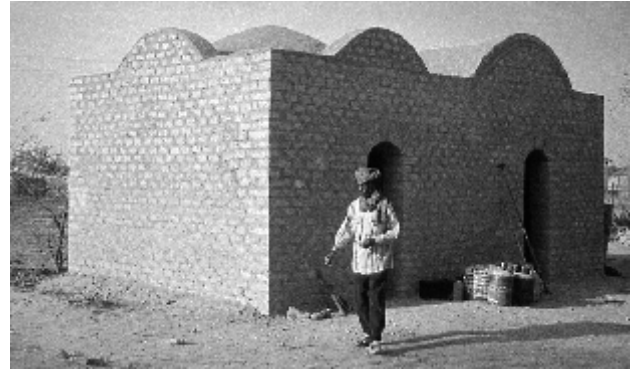
Fig. 12 A small two-roomed house, with one domed room and one vaulted room, provides a good training module.
