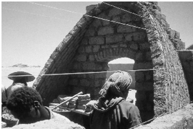
Fig. 5 Starting building out the vault from the end wall.
