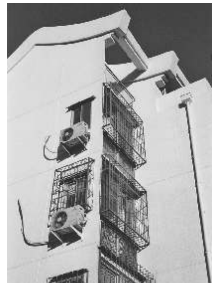
Figure 14 New multi-storey building in Beijing. Comfort and safety are high priority.
