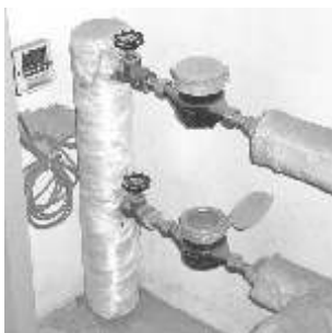
Figure 27 Heating meters.
