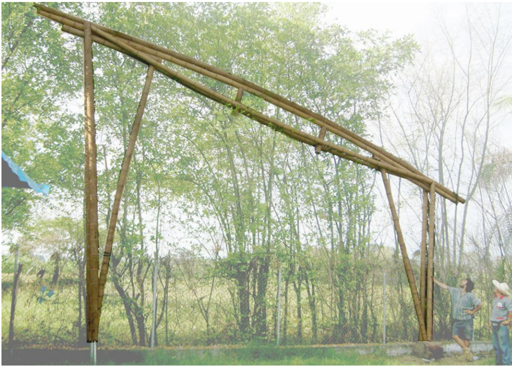
Figure 3: 'Fish truss' by Jörg Stamm. Photograph by the author. Ecobamboo workshop. Colombia, 2009.
