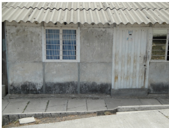
Figure 8. Second housing typology where the construction system is precast concrete panels and light metal profiles which is not suitable for incremental growth and self-construction of a second storey. Photo: Ivette Arroyo, 2009
