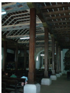
The electric lights are attached to the tie beams over the main nave
