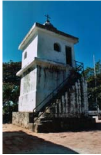
Damage to the belltower
