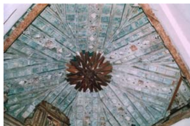
The wooden vault that covers the apse
