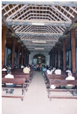
Wooden vaults and ties beams
