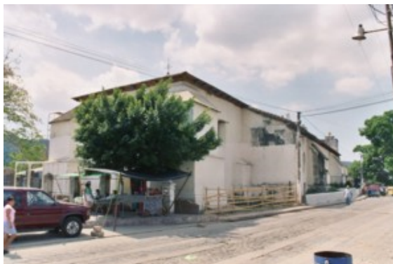
A tree has grown next to the rear or north facade
