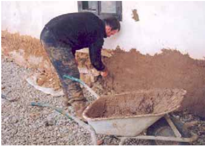
Fig.13 Conservation works of mending the plinth's mortar
