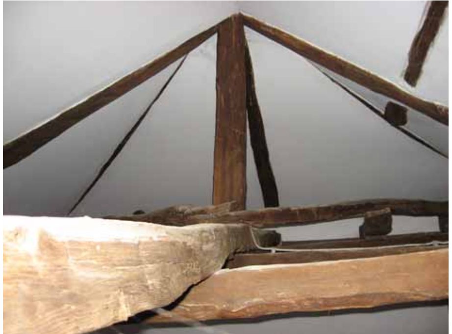
Fig.21 The visible roof system of the stable
