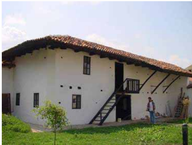
Fig.9 The view of the Stable building
