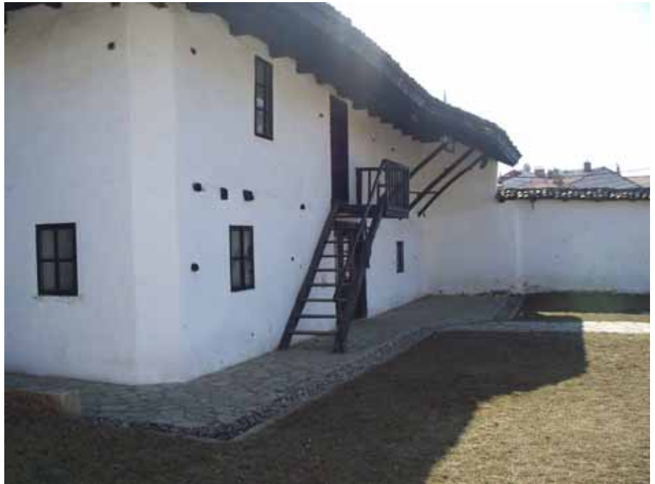
Fig.18 The view of the Stable after the completion of conservation works
