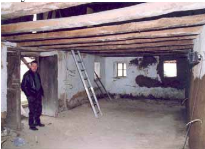
Fig.14 The view of the interior of Stable during conservation
