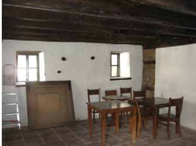
Fig.15 The interior of the Stable after the completion of conservation works
