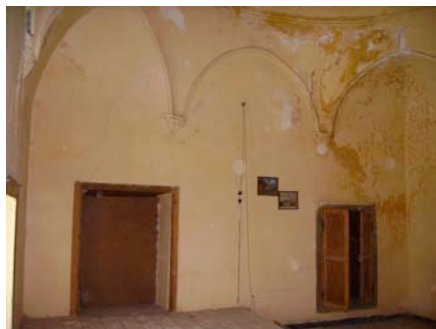
First floor, East view
