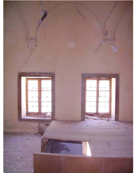
First floor, North view
