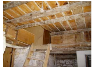
Ground floor ceiling Entrance to first floor
