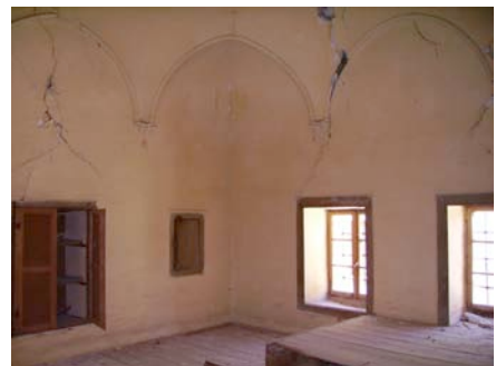
First floor, South-west view
