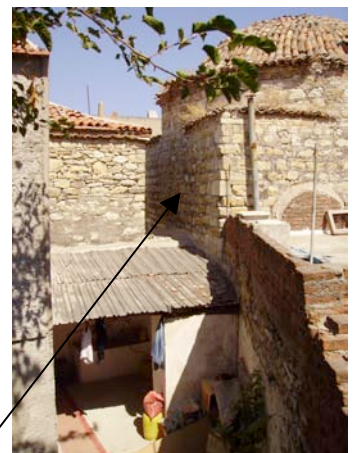
South West view
