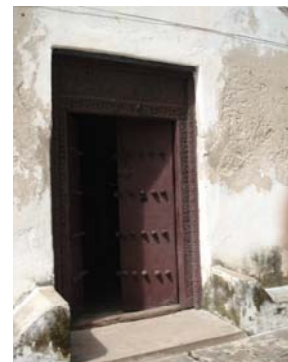
Main entrance door.
