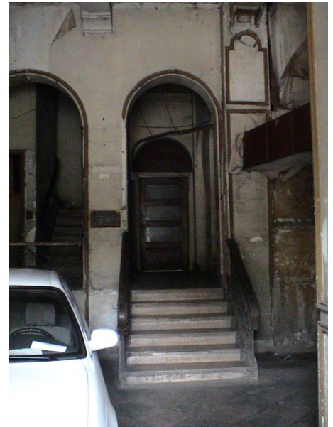
Fig. 22 Elevator Lobby staircase
