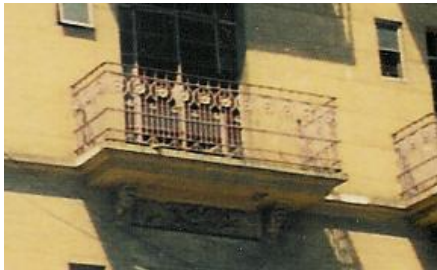
Fig. 17 Grillwork for 3 rd floor balcony
