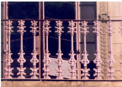
Fig. 18 Grillwork for 4 th floor balcony
