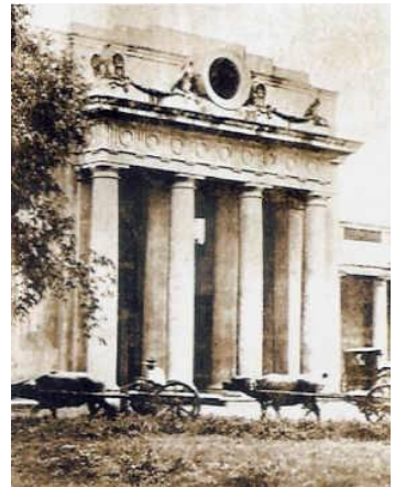
Fig. 5 Paco Train Station
