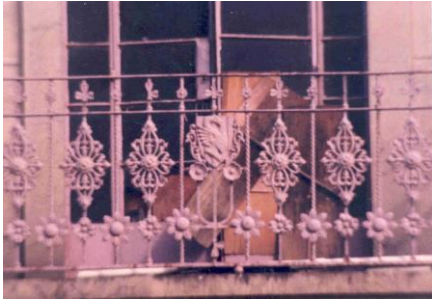
Fig. 16 Grillwork for 2 nd floor balcony
