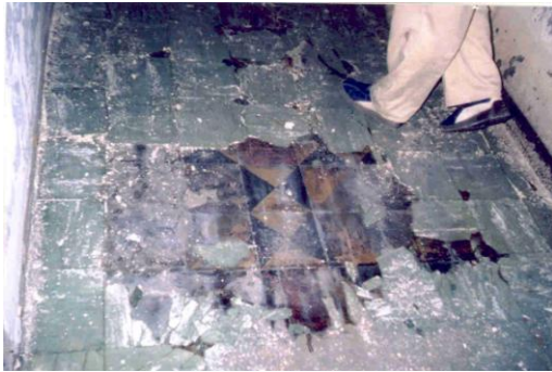
Fig. 30 Original Cement Tiles at Hallway
