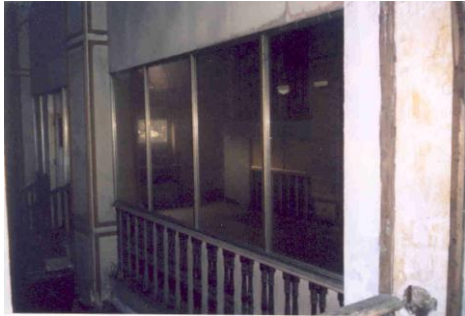
Fig. 19 Elevated Lobby Restaurant
