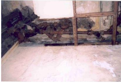
Fig. 29 Drop Ceiling covering plumbing installation.
