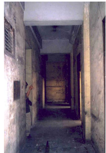
Fig. 25 Hallway along the 2 nd Floor
