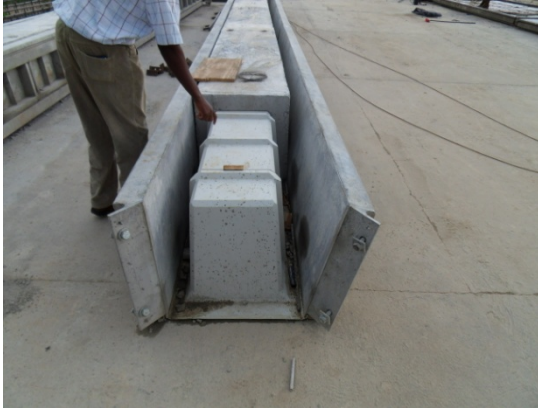
A Reinforced concrete column being moulded
