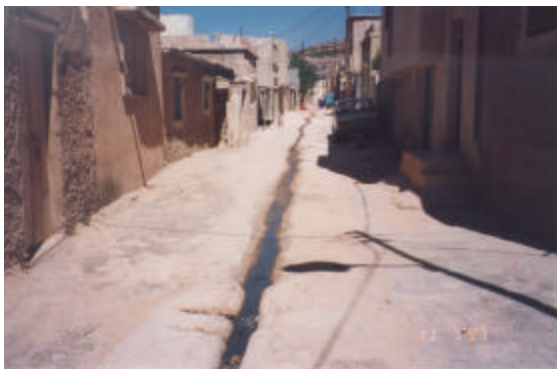
Figure 2 Wastewater floating down the clay roads in Jerash Camp
