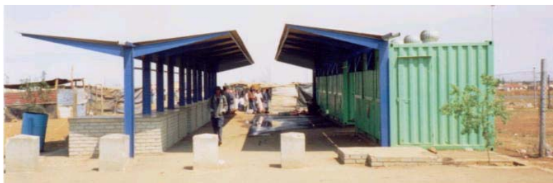
Figure 6 : The completed market structures at Stretford South Entry.
