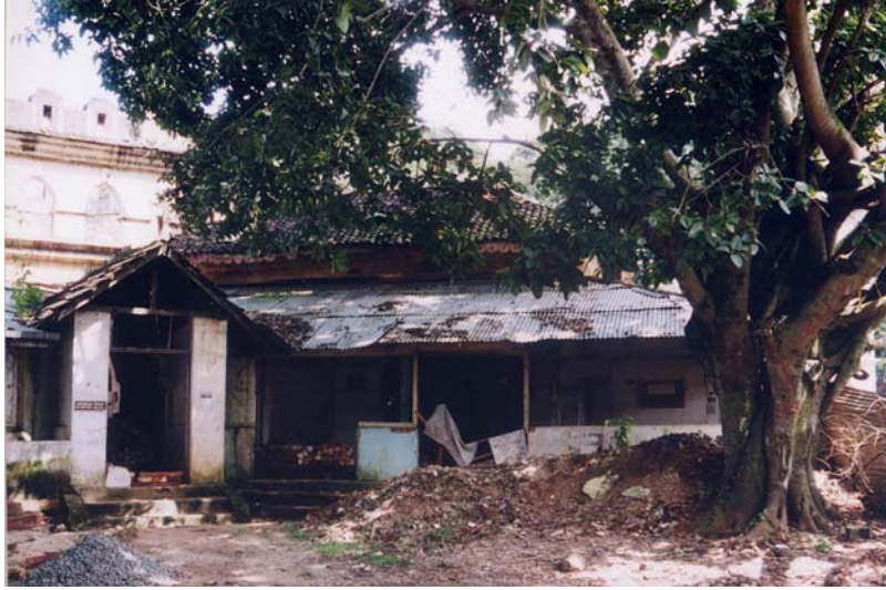
Building with changes for shops
