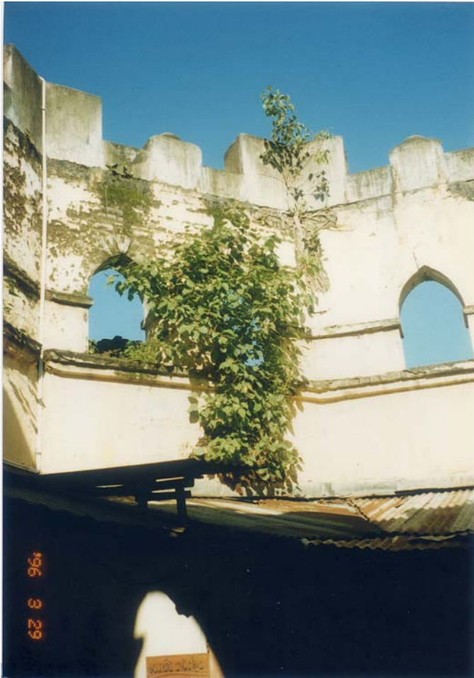
Inner portion of the building without the roof structure
