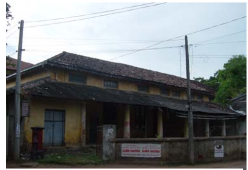
Fig. 20. The Dutch administrative buildings
