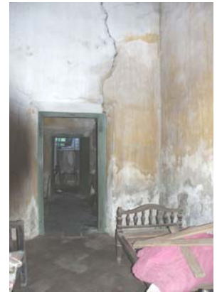
Fig. 38. Cracks infilled.
