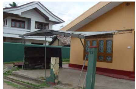
Fig. 33. The Modern house at the rear.
