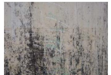
Fig. 39. Damaged plaster.
