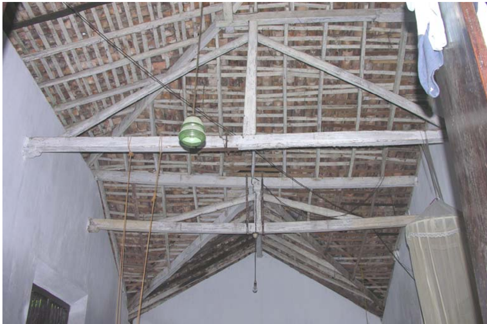
Interior roof structure
