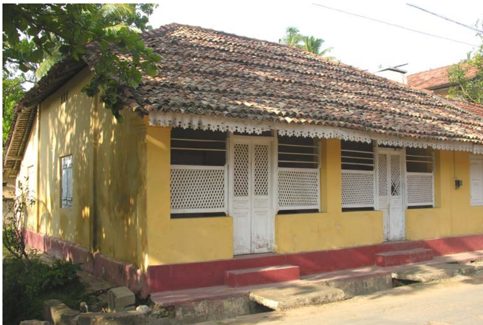
Front view of the building
