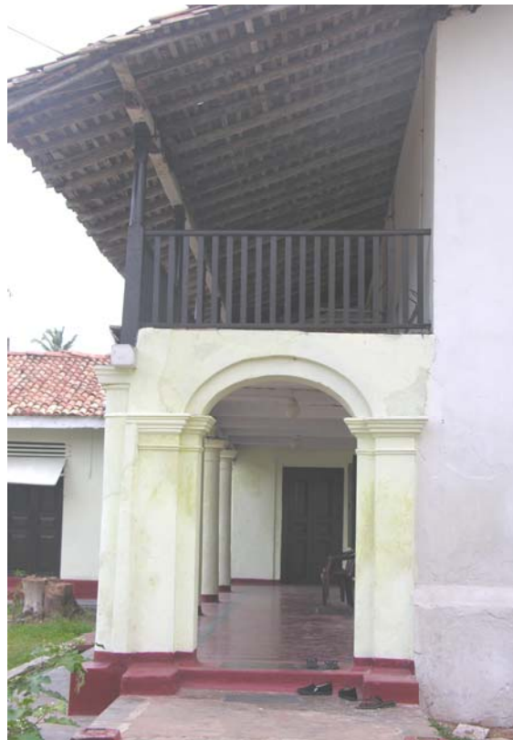
Front view of the house showing the open verandah, wooden balcony with timber railing and pillar and the tiled gable roof
