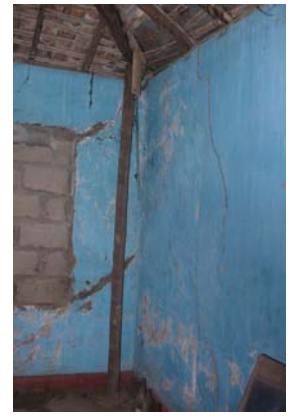
Fig. 37. Timber propos are used to stabiles the roof.
