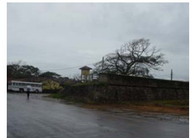
Fig. 12 The south bastion demolished.
