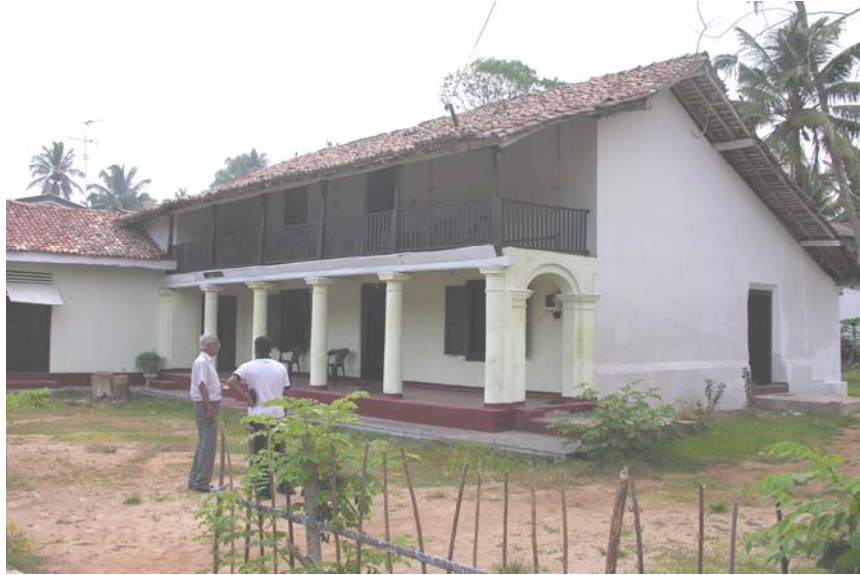
Front view of the house showing the open verandah, wooden balcony with timber railing and pillar and the tiled gable roof
