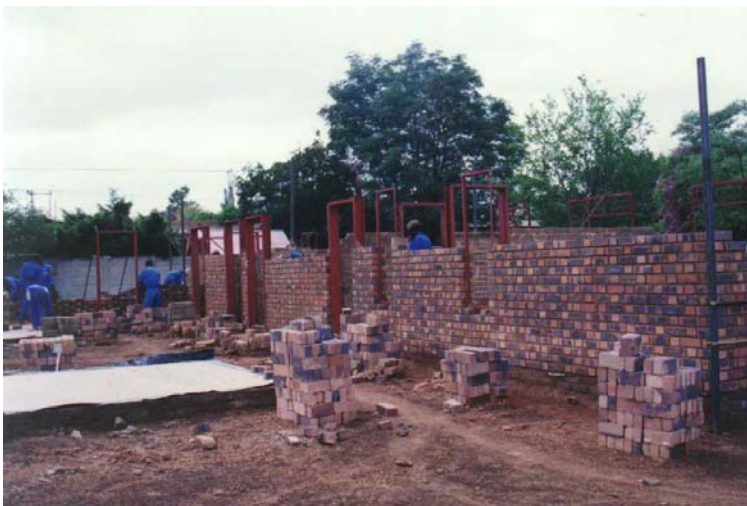
Picture 1. The bricklayers are putting up part of the walls.
