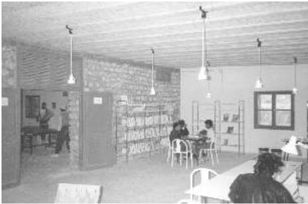
Fig. 44 The roof in Fig. 41 as built in the youth centre of Tameghza, Southern Tunisia. Woodwool slabs provide both thermal insulation and sound absorption.
