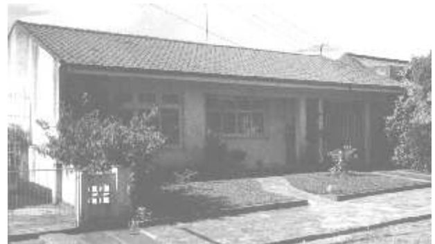
Fig. 37 Above: House in Porto Alegre, Brazil, built with the “Climatex system” (Fig. 36) with prefabricated wall elements of woodwool slabs and concrete.
