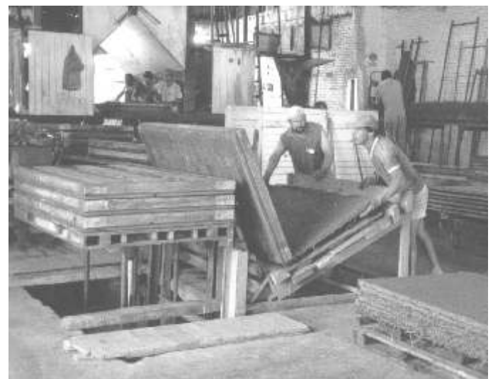
Fig. 18 Stripping 24 hour old slabs (Climatex, Brazil).
