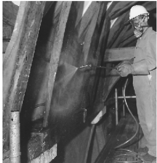
Figure 2 shows the personal protective equipment necessary when spraying a solvent-borne insecticide in a roof space.
