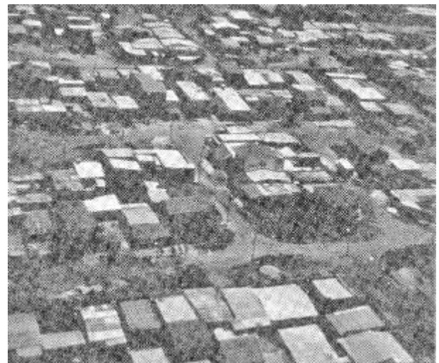
Low income incremental land development scheme, low rise, high density. Satellite city of Samambaia, Brasilia.
