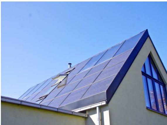
Figure 3: A well-integrated solution, +energy house in Åkarp 23
