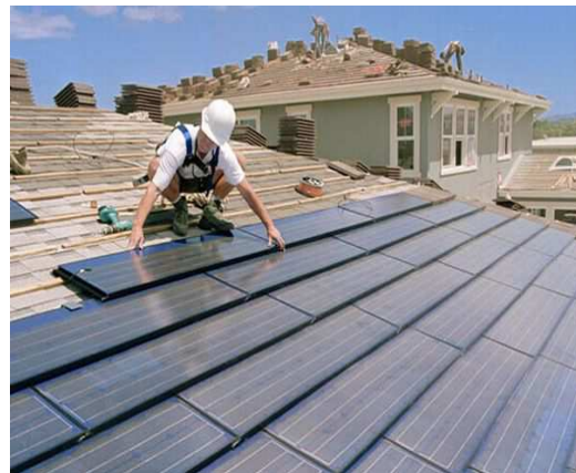
Figure 4: PVs as roofing material 24
