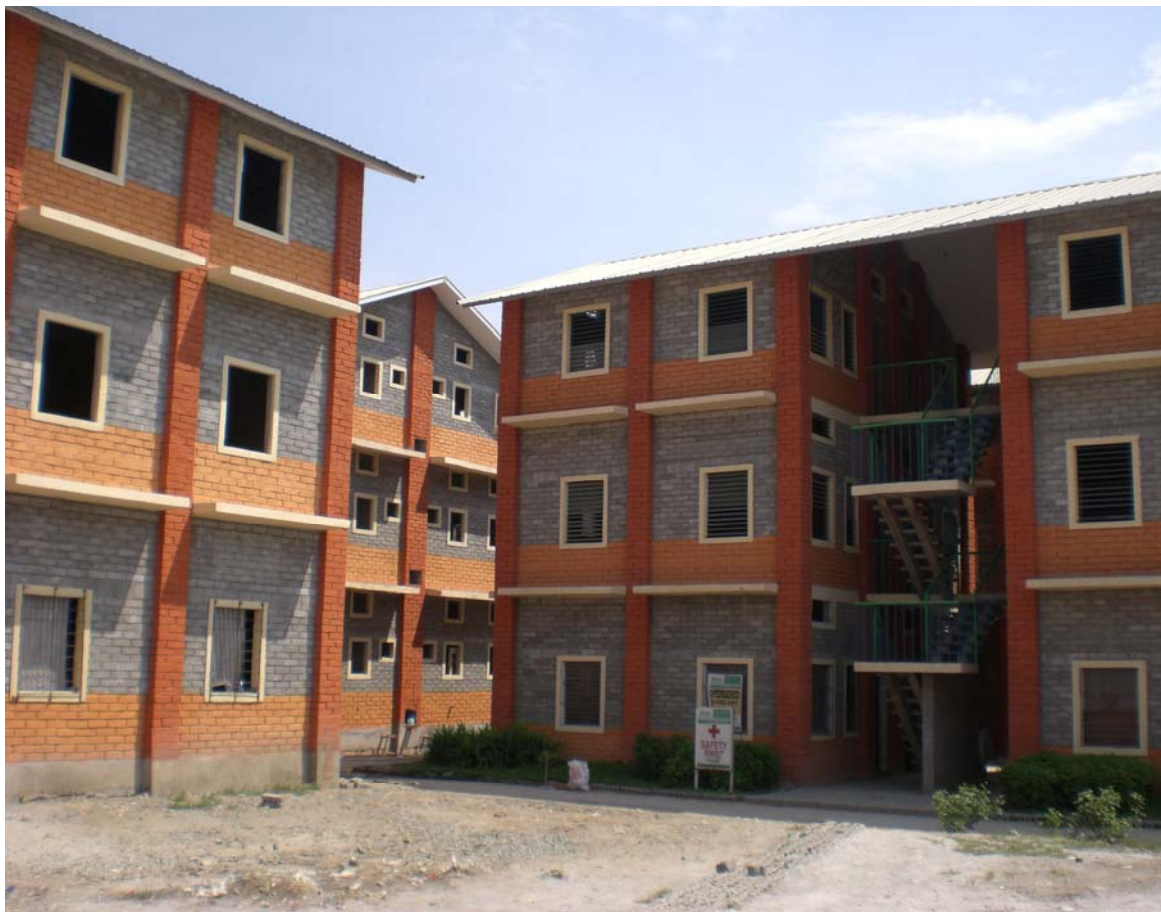
Fig 16. Medium-rise buildings by HfH in Taguig built with interlocking concrete blocks. Lofts can be installed in all condominiums, making the houses taller than normal three storey buildings.
