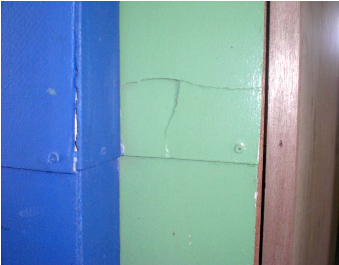
Fig 31. A crack in the wall of a HfH house shows how brittle the cement fiber boards used here are.
