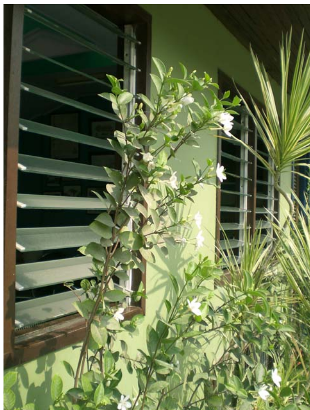
Fig 32. Louver windows give good airflow.
