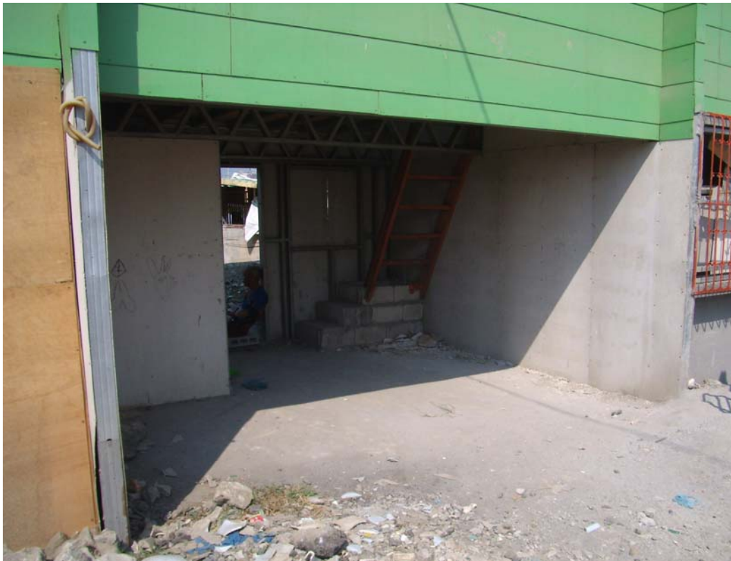
Fig 29. This HfH building shows the foundations lack of elevation
