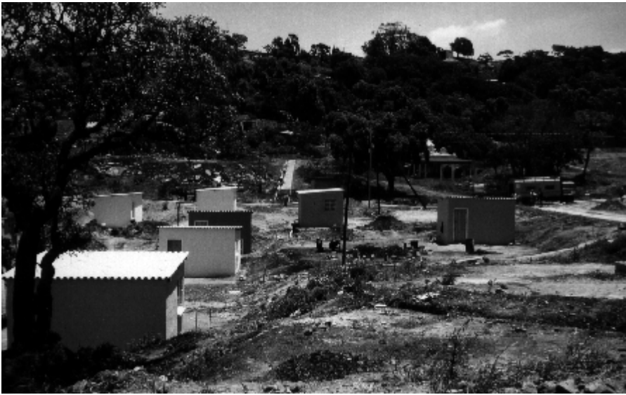
New houses in Wiggins Umkumbane, Cato Manor. One of several housing projects developed and managed by CMDA.
