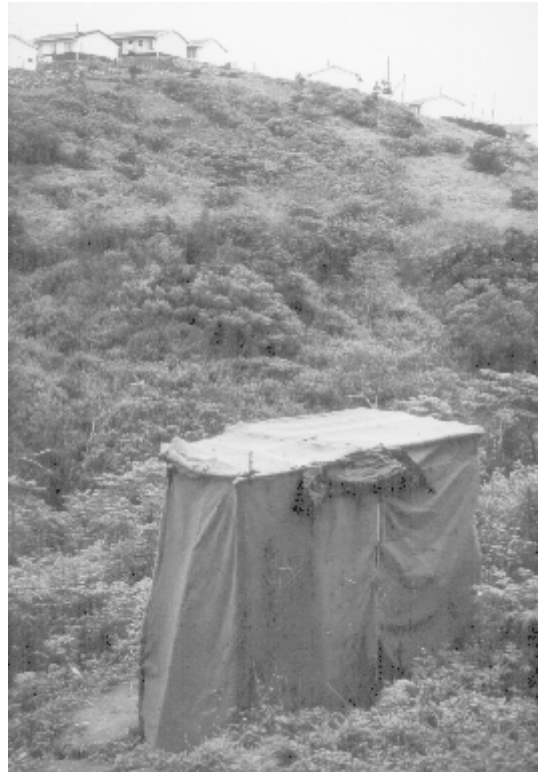
The pit latrine is often situated at the far end of the plot and surrounded by lush vegetation.
