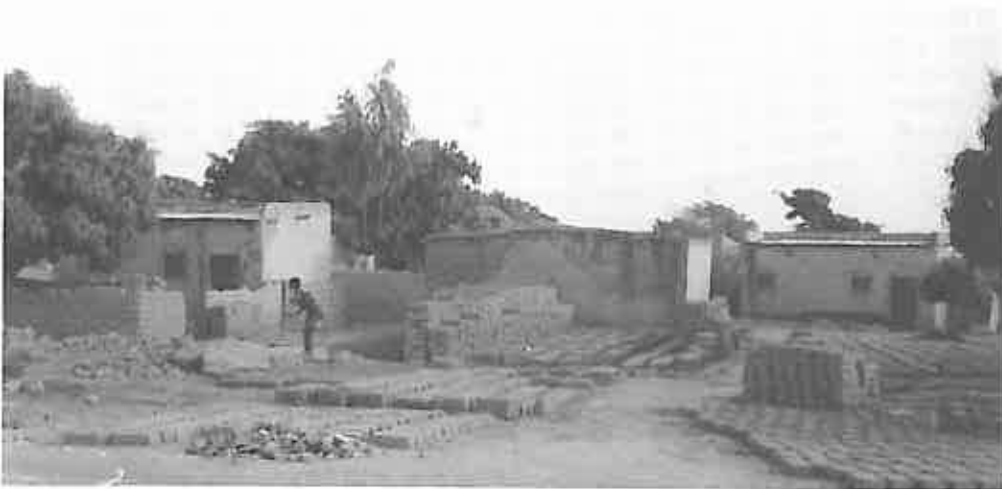
Storage of adobe blocks
