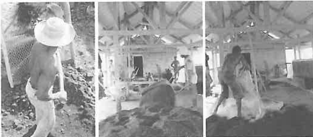
Making stabilized earth blocks.
