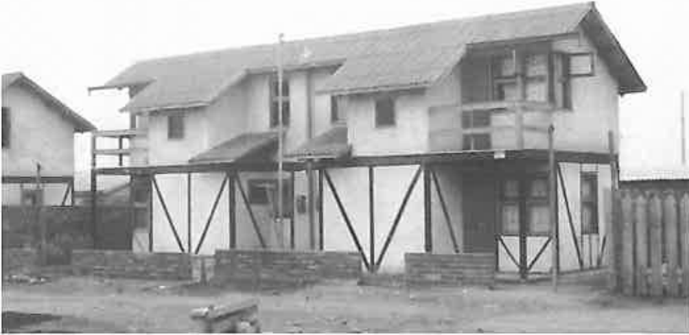
Wood-frame housing construction.
