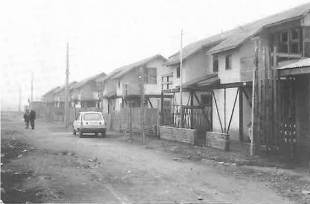
Newly-built housing with stabilized earth.
