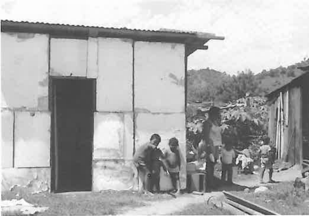
Housing completed with wall section.
