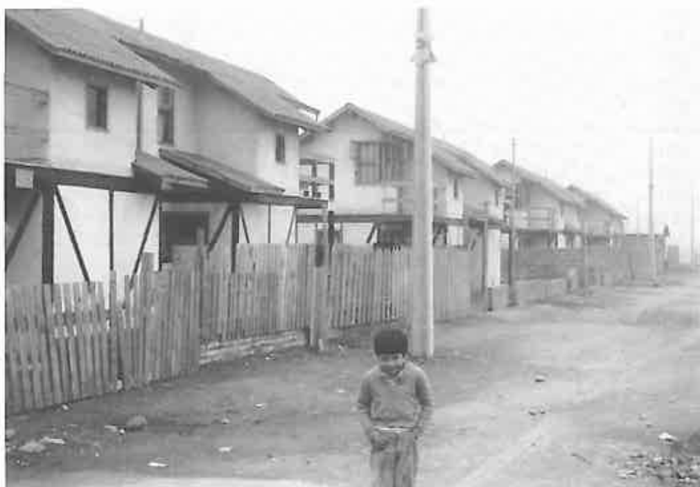
Newly-built housing with stabilized earth.
