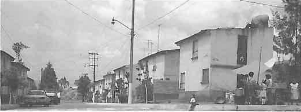
Basic infrastructure is installed and the streets paved.
