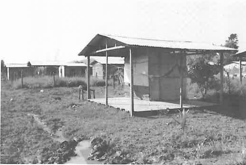
Newly-built housing frame with roofing.
