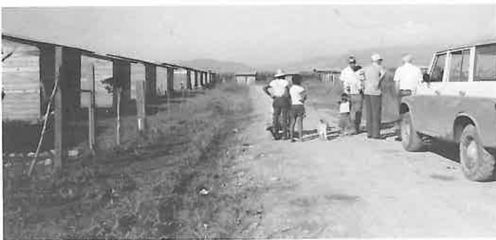
View of a completed housing area.
