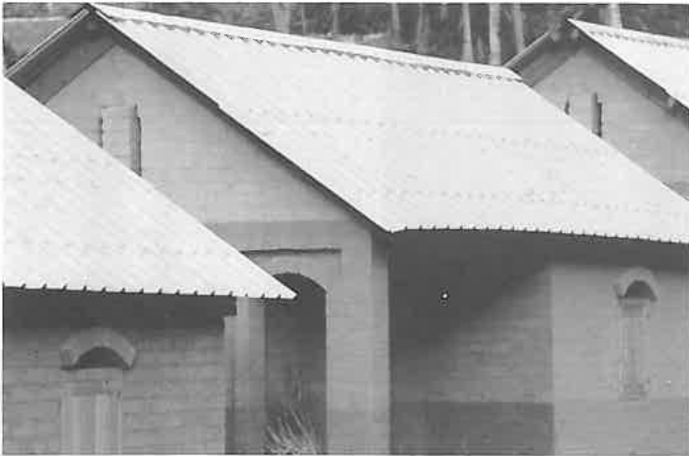
Newly-built housing of stabilized earth blocks.
