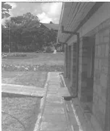
Long overhangs and hard paving against the building protect it from rain
