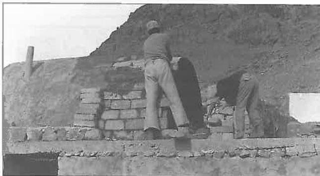
Building a vault roof with cement stabilized earth blocks, Tunisia
