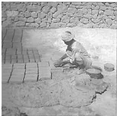
Moulding clay bricks by hand
