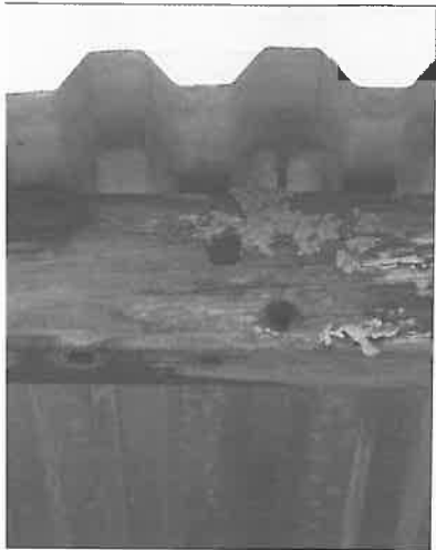
Holes in a timber beam caused by bumble-bees
