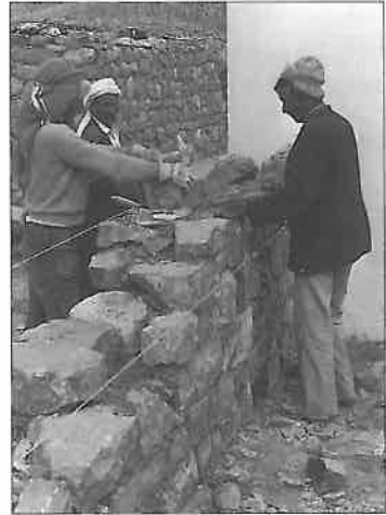
Laying a stone wall
