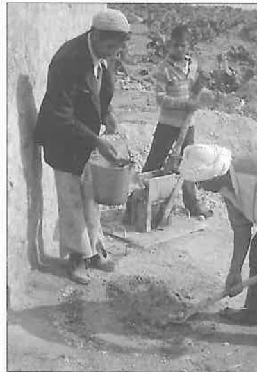
Making cement stabilized earth/soil blocks
