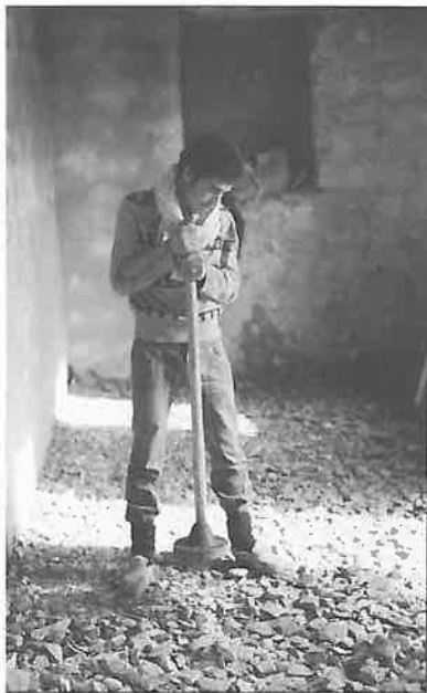
Compacting the gravel before casting a concrete floor.
