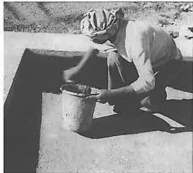
Laying a waterproofing membrane on a flat roof.
