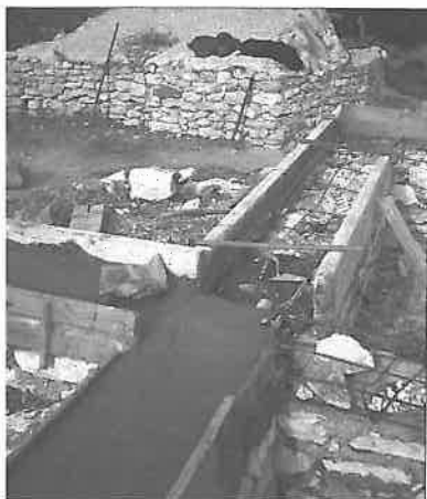
Casting the strip footing.
