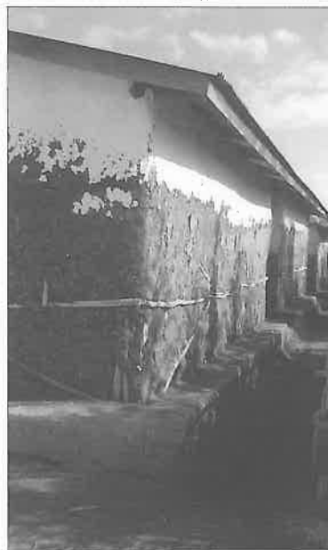
A problem with lime paint is that it washes away in rain.
