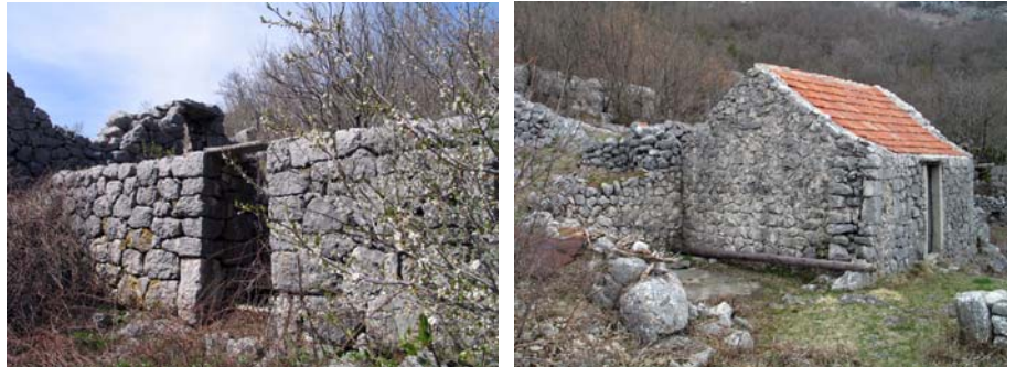
Figure 9 | The site – the older and the newer house
