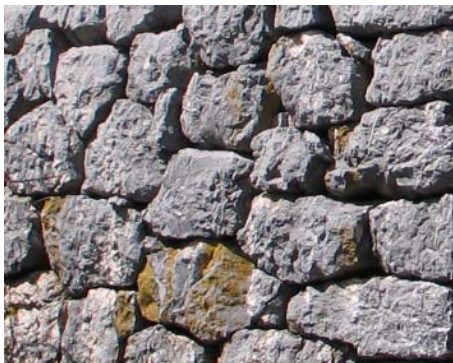
Figure 11 | The dry stone wall
