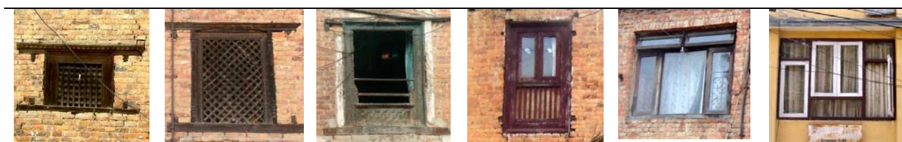
[b] Modification of window opening
