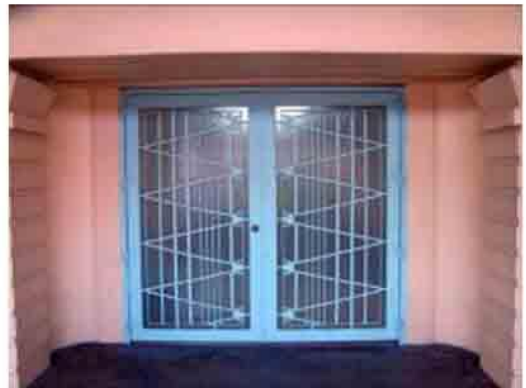
Photo 76. The main entrance door (center) at NRH facade is no longer being used for access. Accent lighting should be placed.
