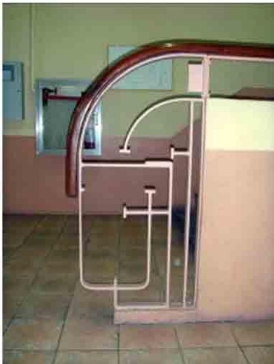
Photo 11. Art Deco stair railing designed with the initials "FEU". Wall at background installed externally with a fire hose rack and fire alarm annunciator. Needs refurbishing.
