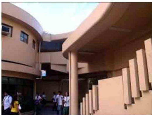
Photo 3. Art Deco stair leads to 2nd floor. A bridge way connects NRH to Science Building. This connection should have aesthetic elements to show transition from the old building to the next building.
