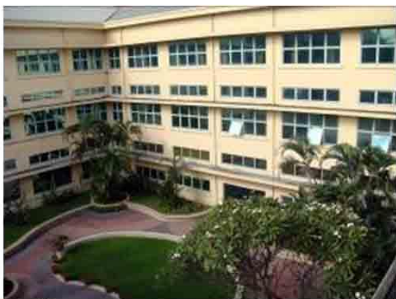
Photo 66. Another view of the commemorative garden showing left right wing of building and middle section of NRH. Note partially opened awning windows which cannot be closed because of protruding WACUs.
