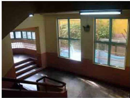
Photo 34. The stairway landing leads to the bridge way
