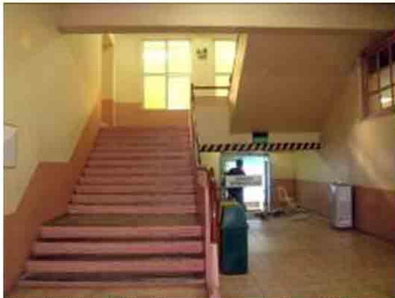
Photo 10. Original right side main stairway leads to 2F. Note character of old high wood casement glass window to that of the new one installed one at the stairway landing
