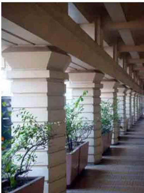
Photo 74. The arcade with original Art Deco columns and original tile flooring
