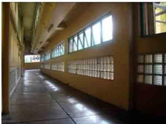
Photo 37. The bridge way with original flooring, glass blocks, and with newly installed awing glass windows
