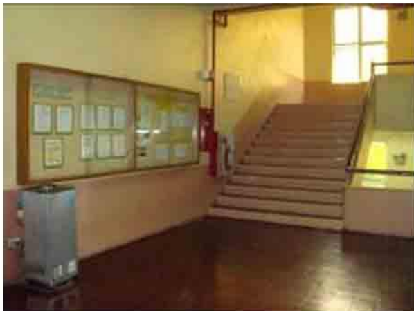
Photo 41. Right wing stairway leads to 3F. Note of the presence of utility pipes (fire sprinkler) for fire mitigation.
