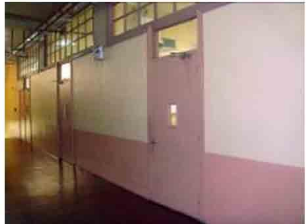
Photo 44. The original wall character of the classrooms showing original doors and high windows. Should be preserved.
