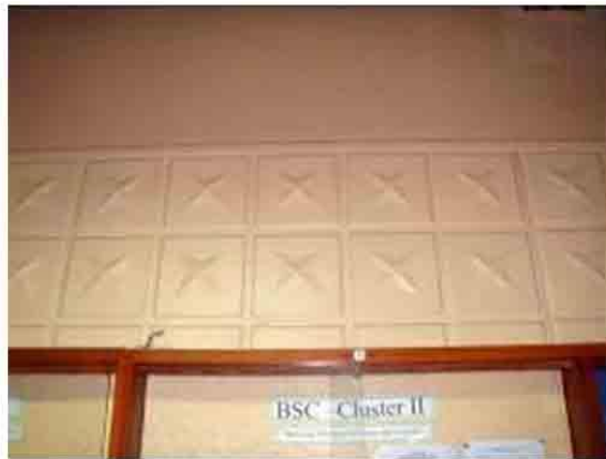
Photo 23. Original Art Deco wall artwork near Study Area. Should be preserved.
