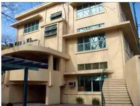
Photo 56. NRH right wing external character. Stairway at right is leads to the grandstand where student programs are held.
