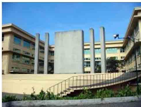
Photo 58. NRH Rear Elevation shows the symmetrical U-shape form of the building.
