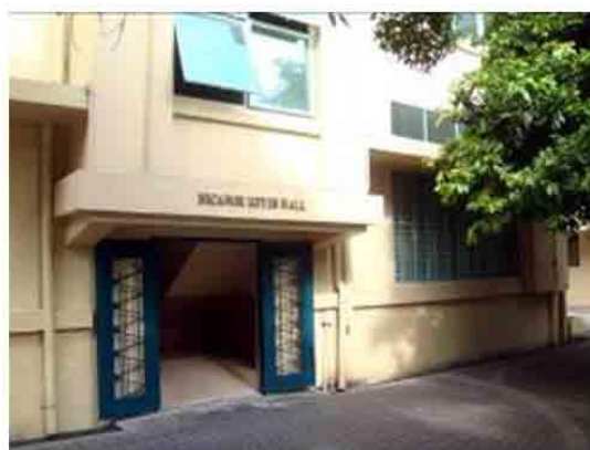
Photo 59. The rear entrance at the left wing of NRH. This is where the signage-name of the building is placed. Should be placed at a more emphasized location.
