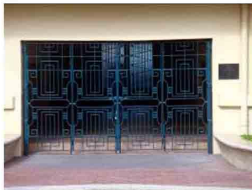
Photo 63. Art Deco steel grille door at middle section of NRH serves for an occasional entrance. UNESCO marker is placed at the right side adjacent to an exposed downspout
