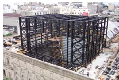
Figure 13: Rehabilitation Works, the new structure of the Stage, 2003.
