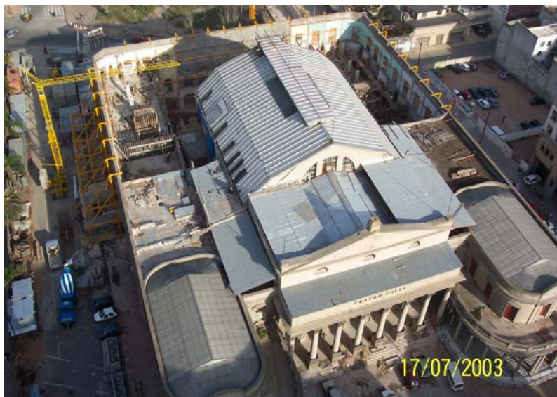
Figure 12: Rehabilitation Works, the Stage and Lateral Wings demolished, 2003.
