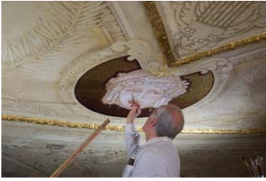
Figure 15: Rehabilitation Works, the Plafond Restoration, 2003.
