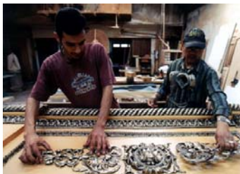
Figure 20: Rehabilitation Works, the Front boxes Restoration, 2003.
