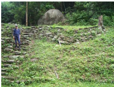
Figure 16. Sinking due to settlement of land.
