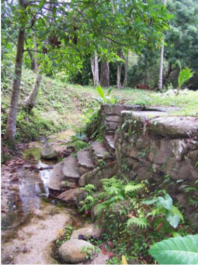
Figure 9. A slope is cut to make a cross section. Stair with access to the river
