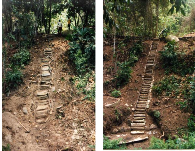
Figure 6. Cadavid photos of phase II (1988) before and after the intervention.
