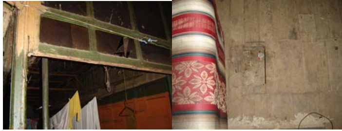
Left: Courtyard Covered , Right: Damaged part of the Parquet floor
