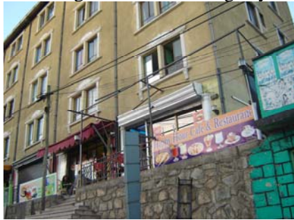
Figure 5: facade decoration on a low cost apartment close to the house
