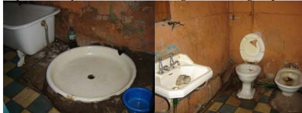
Sanitary fixtures to be replace and mended in the bath rooms
