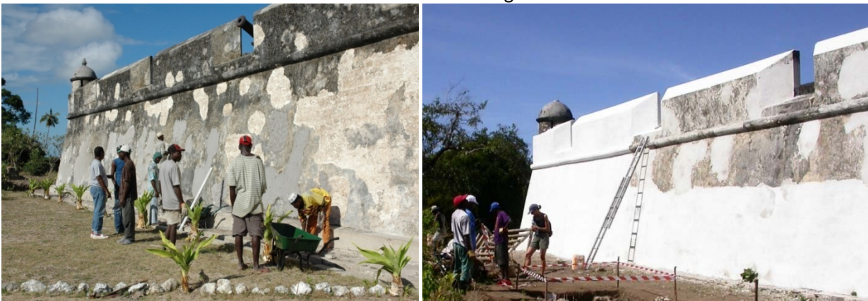
Repair works on external wall
