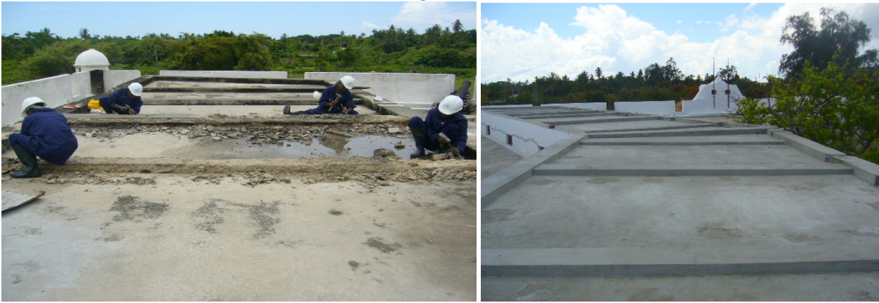
The Flat concrete roof - the intervention
