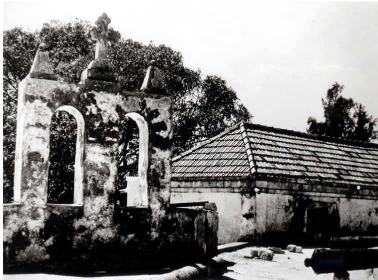
At one time, the building had a double pitched clay tile roof. (Credit)
