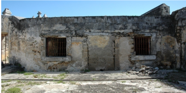
Elevation of the Kitchen from the Courtyard (With Sealed Doorway) April 2006.
