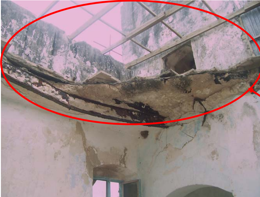
Figure 15: Part of Collapsed Flat Roof
