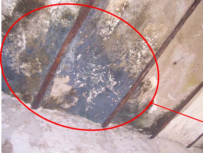
Figure 11: Condensation and black mould and stains growth on the walls and slabs
