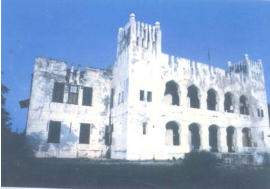
Figure 2: Front View of the Old Boma before the collapse of the Balcony
