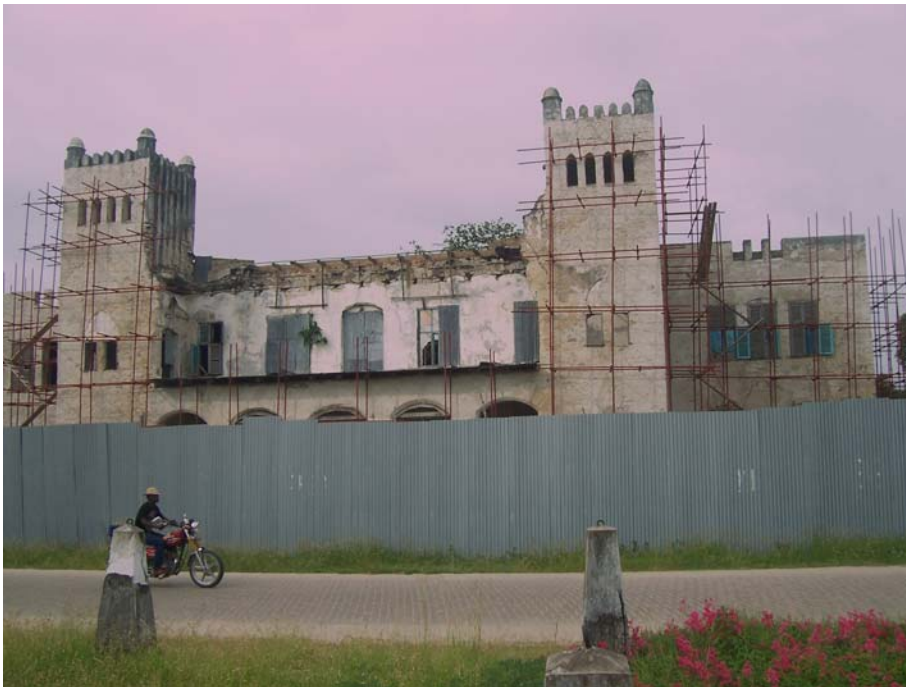
Figure 9: Front View of the Boma – Current situation
