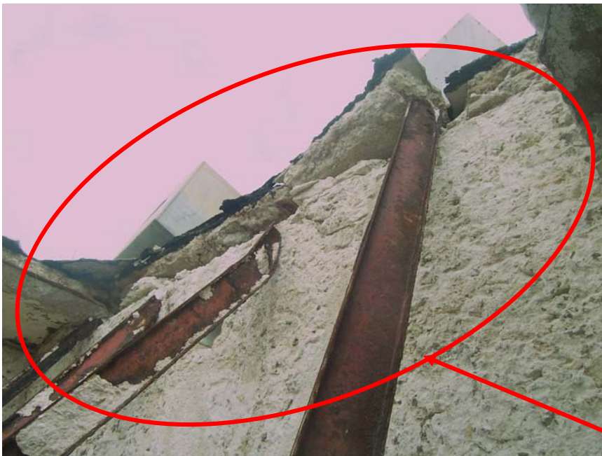
Figure 14: Part of collapsed Roof exposing corroded I-beams
