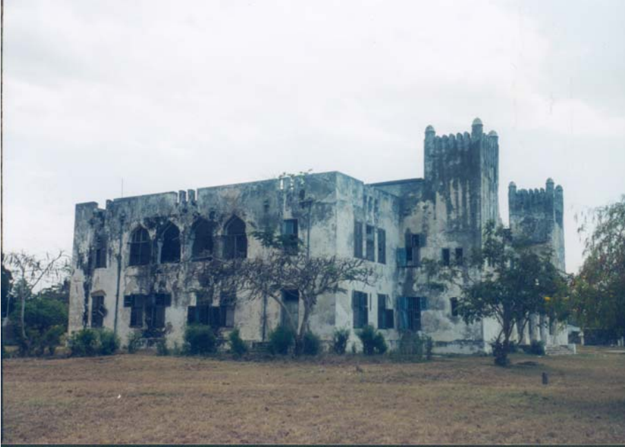
Figure 4: Left Side View of the Old Boma before the collapse of the Balcony
