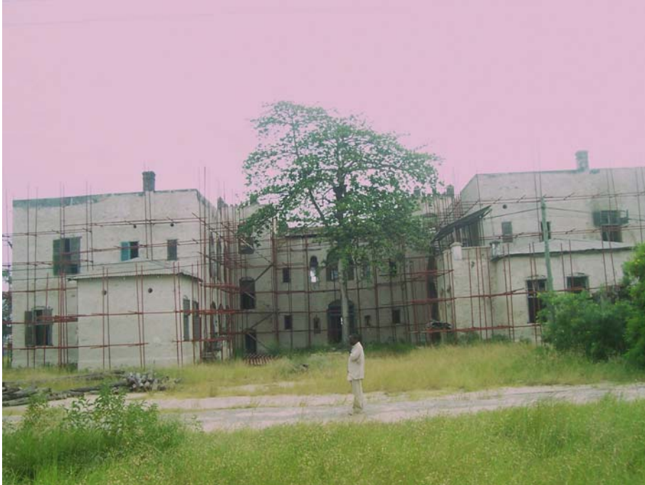
Figure 10: Rear View of the Boma – Current situation
