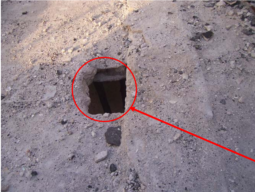
Figure 13: Damaged Floor with the Through Hole
