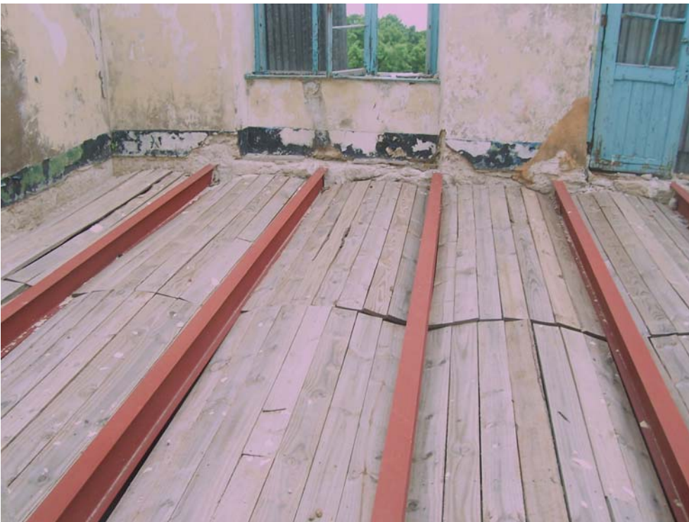
Figure 18: Part of the upper floor slab completely under restoration
