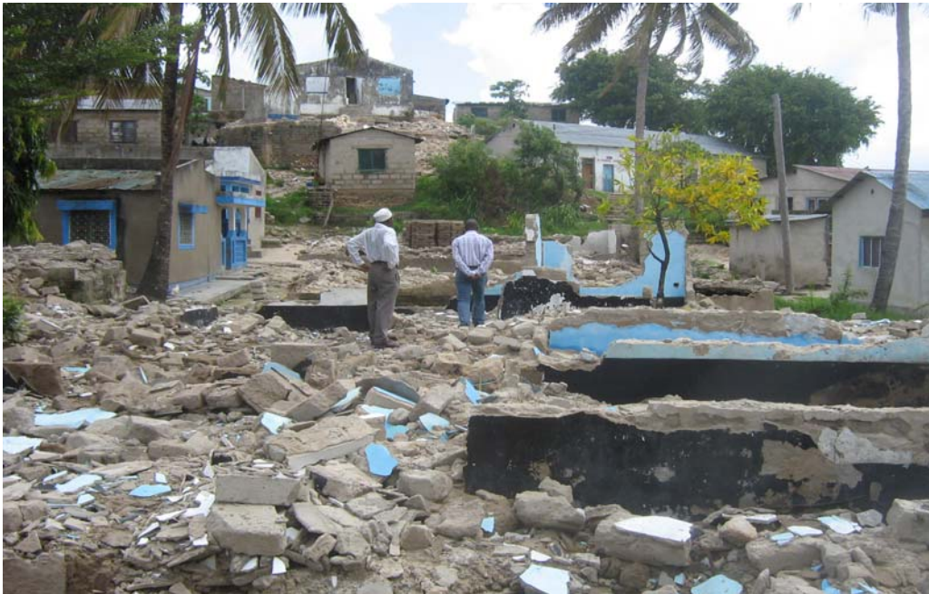
Fig 2. Demolition of houses in Kurasini Resettlement
