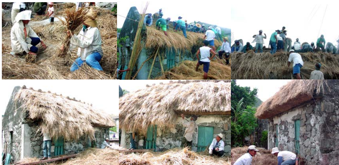
Fig. 19 to 24 – Kamañidungan Cooperative’s Re-Roofing Activity
