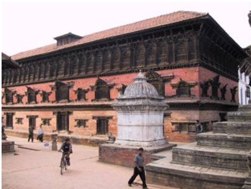
55 WINDOWS PALACE BEFORE RENOVATION
