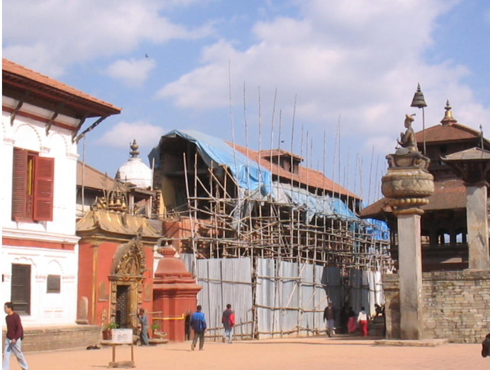
CONSERVATION WORK OF PALACE TOWARDS THIRD PHASE
