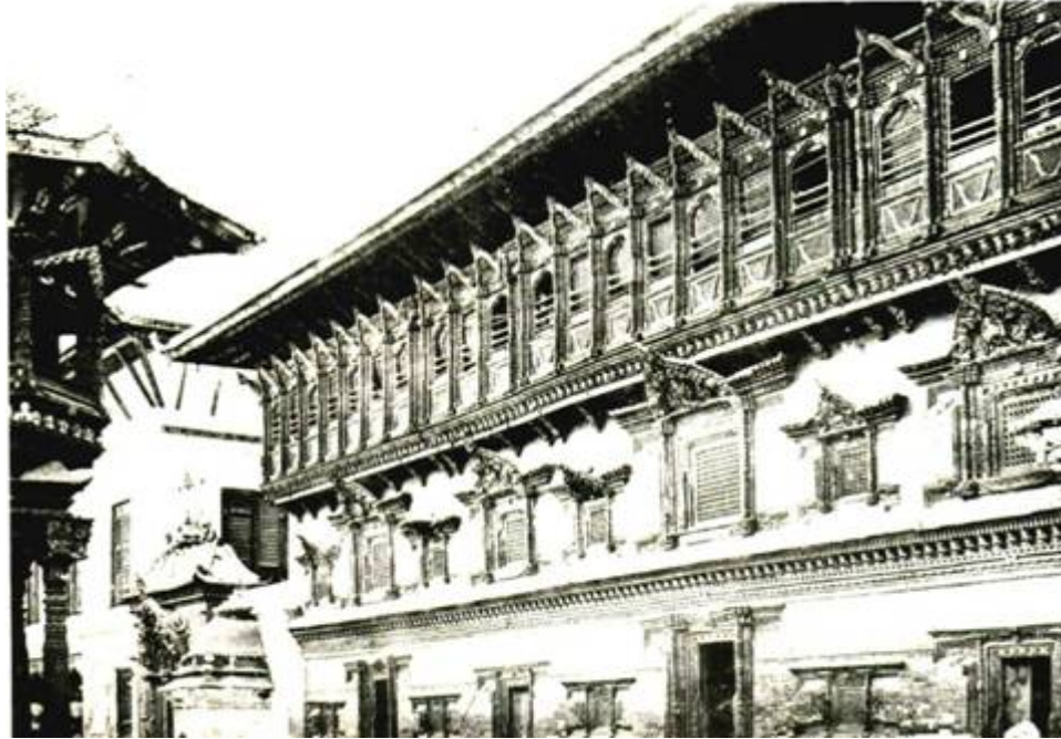
SOUTH-EAST VIEW OF 55 WINDOWS PALACE BEFORE 1934 EARTHQAKE
