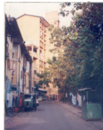
Maligawatte Housing Scheme
