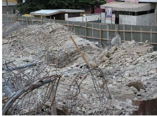
Figure 4. The remains of a four Storey commercial Complex which collapsed during construction. No lives were lost here but the financial losses were close to four hundred thousand Dollars.
