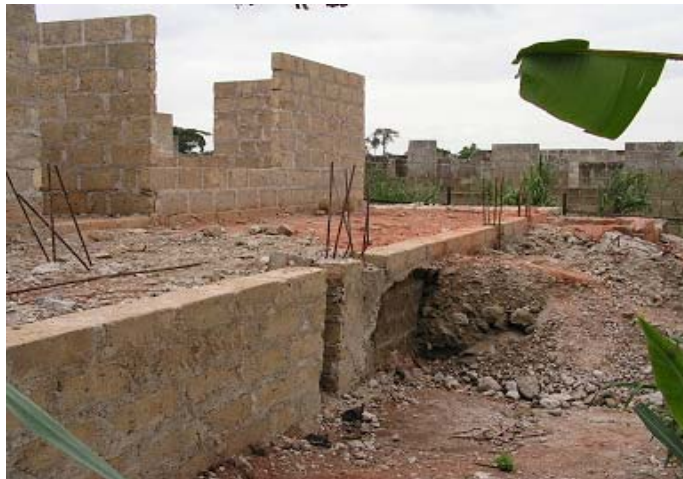
Figure 2.A Two storey domestic building, Roofed and Wired, ready for plastering. This Building failed during a mild Storm. It is now being reconstructed into a single storey building.
