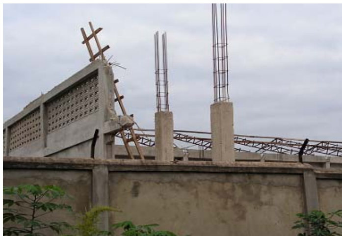
Figure 2.A Two storey domestic building, Roofed and Wired, ready for plastering. This Building failed during a mild Storm. It is now being reconstructed into a single storey building.
