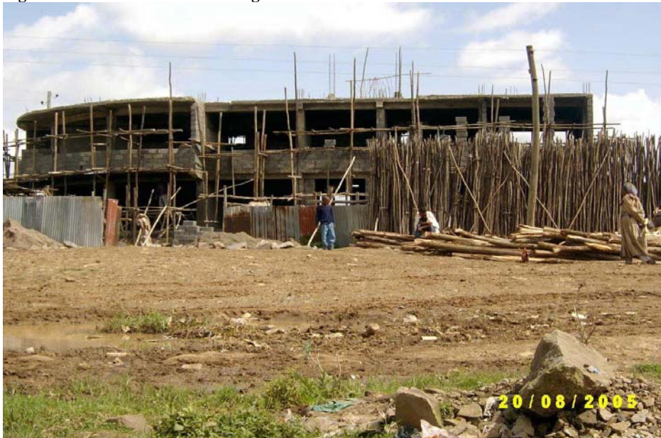
Figure 5.5 Construction of building for business
