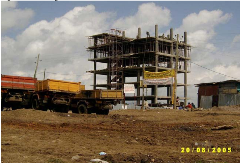
Figure 5.6 Building under construction
